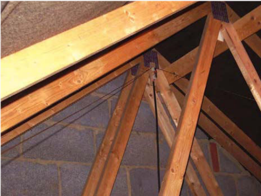
Fig. 7: Looking up into the apex of the roof, showing the inverted-V formed with the wires. The angle formed will most likely be different in house of different ages, as roof apex-angles have changed.
